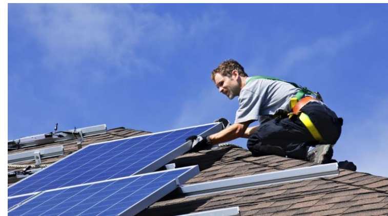
A person installs solar panels on a rooftop.
